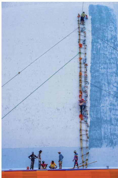
Salon HM - GUIXIANG HUANG, China, External wall plastering
